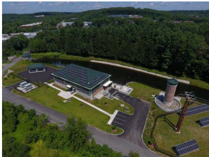
Figure 13: WAPS Geothermal Heat Pump Installation
