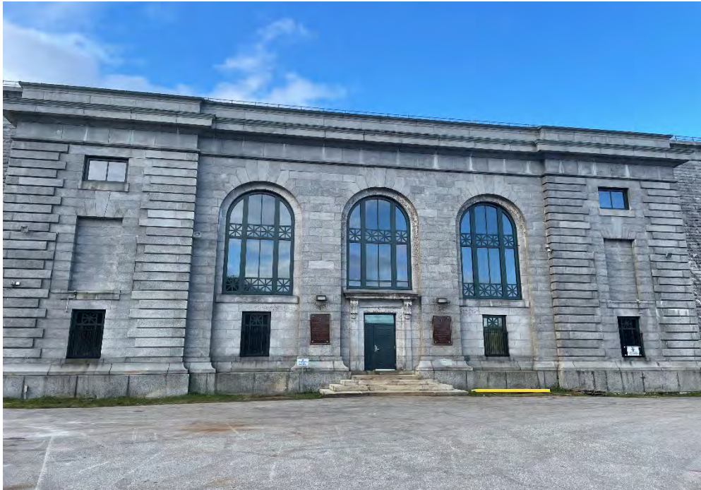
Wachusett Dam Lower Gatehouse
